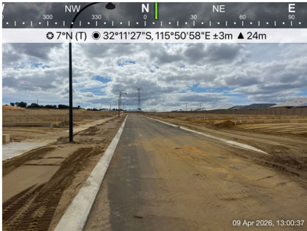
Plate 1: Walker Road within Stage 15B.
