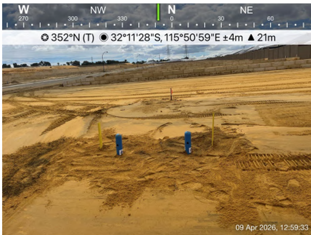
Plate 3: Taps with protectors fitted connected to the reticulated water network within the subject site.
