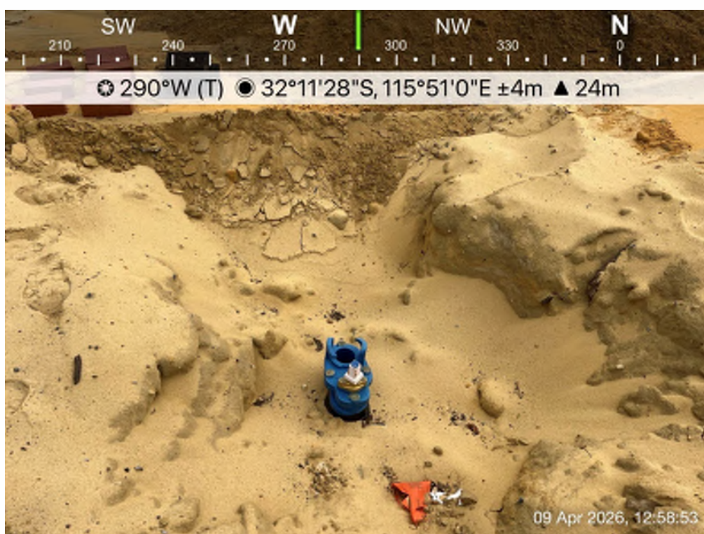
Plate 3: Taps with protectors fitted connected to the reticulated water network within the subject site.
