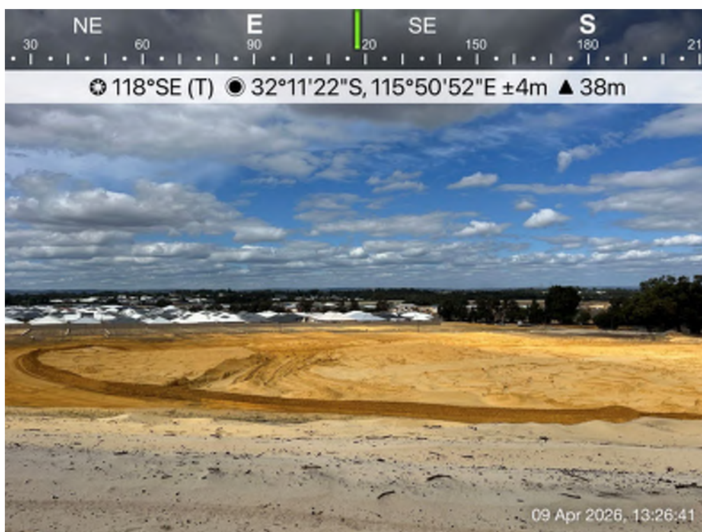
Plate 8: Clearing of Lot 9014
