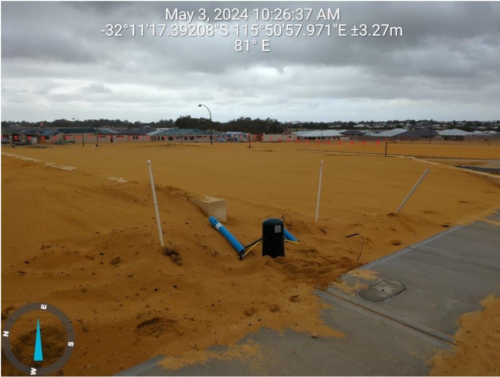
Plate 7: Reticulated water connection throughout Stage 9.
