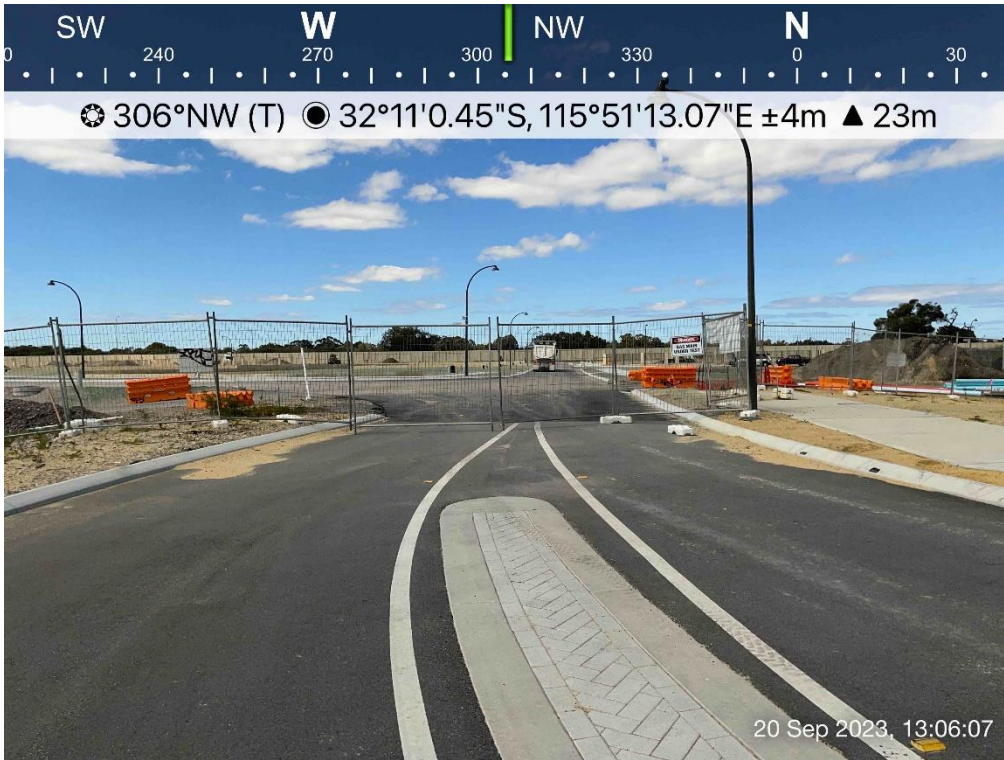
Plate 5: Entrance to Emergency Access Way showing unlocked gates
