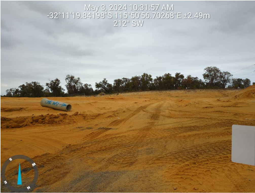
Plate 1: Cleared areas within the subject site and surrounds
