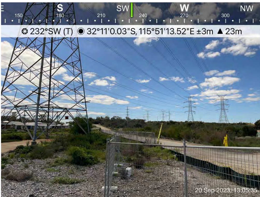
Plate 4: Emergency Access Way
