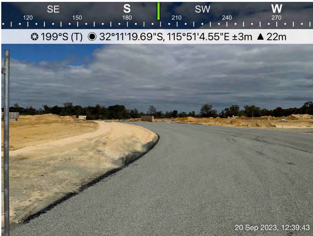
Plate 6: Road under construction within the subject site
