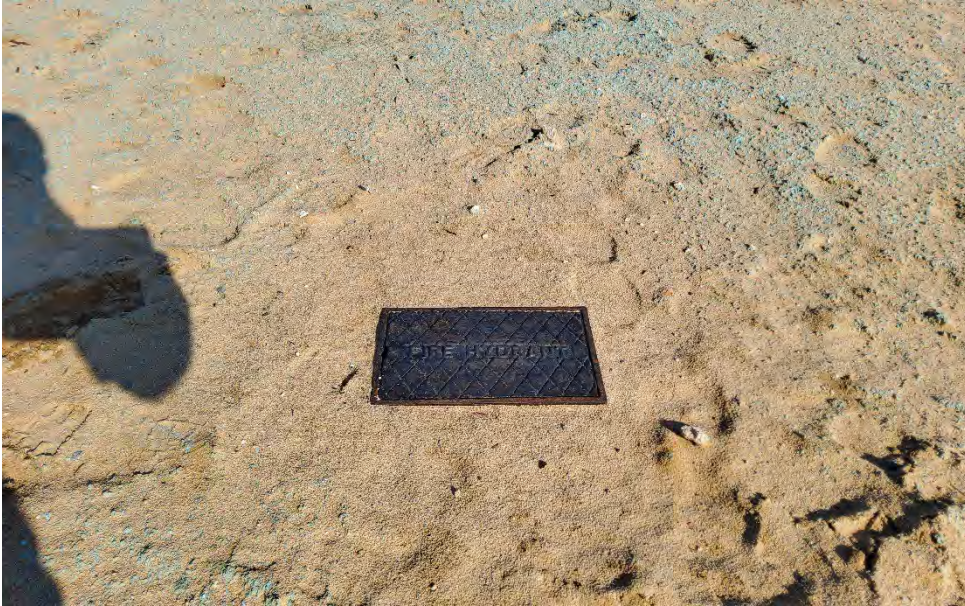
Plate 9: Installation of hydrant within neighbouring Stage 12
