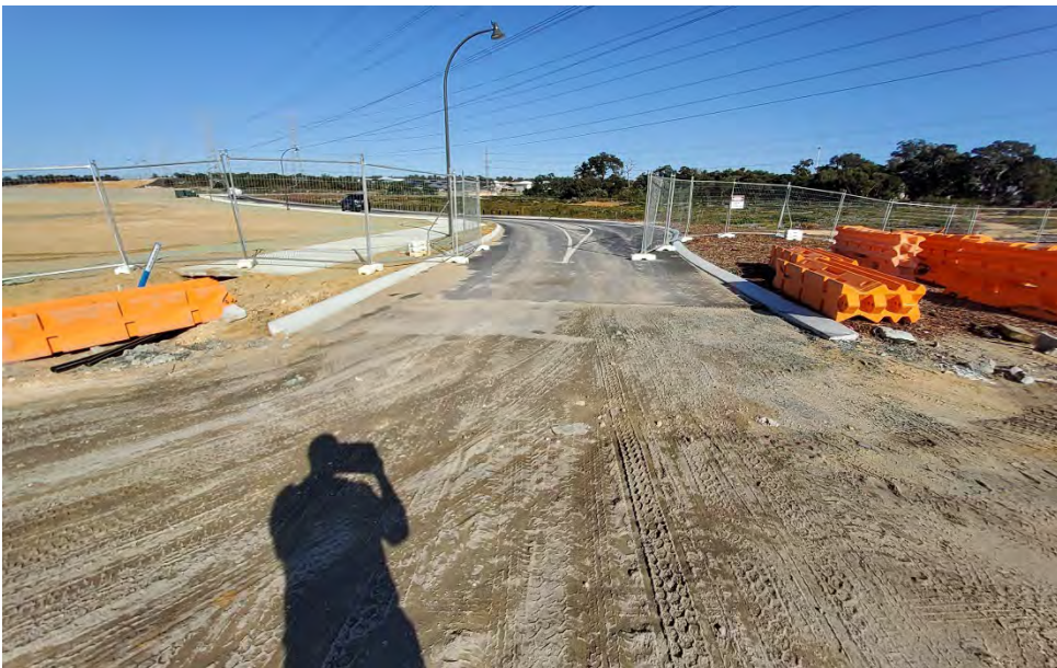
Plate 6: Route to temporary Emergency access way.
