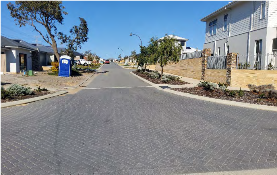
Plate 5: Standard of road and road verge in completed stage nearby.
