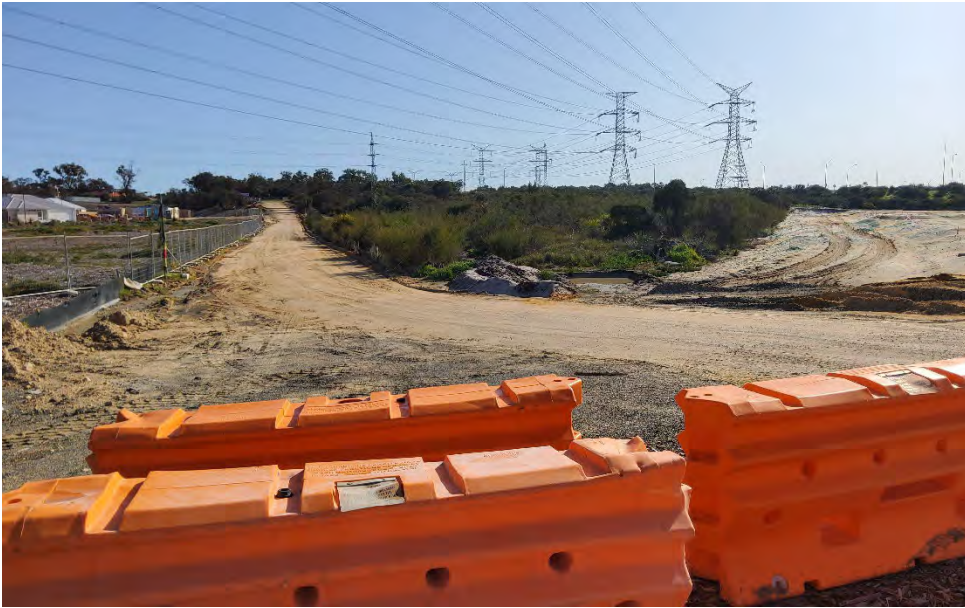
Plate 7: Temporary Emergency access way.
