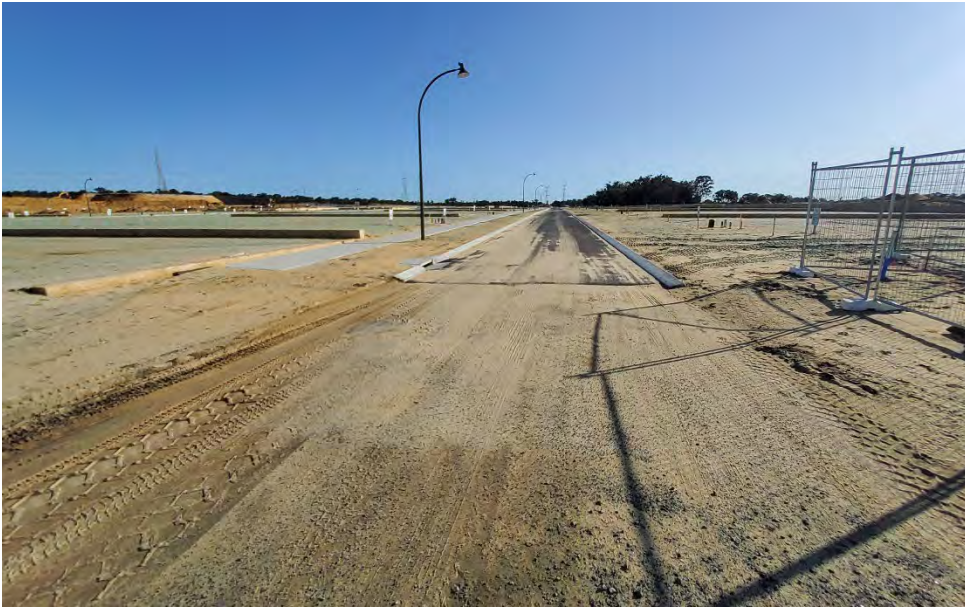
Plate 3: Current condition of road and road verge construction within neighbouring Stage 12.
