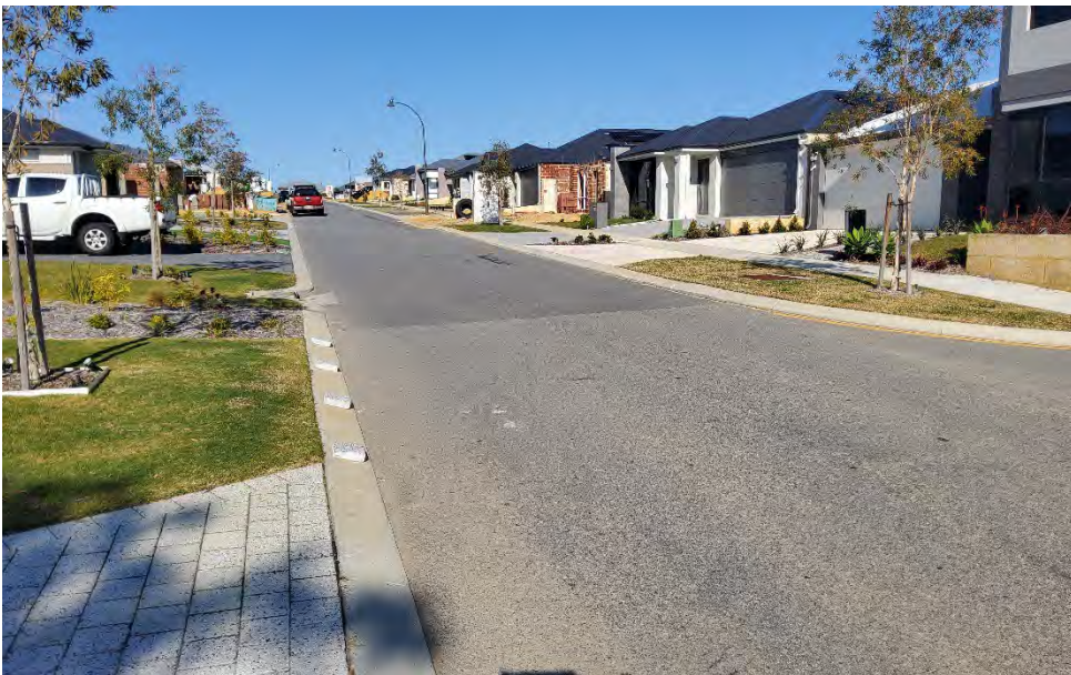
Plate 4: Standard of road and road verge in completed stage nearby.
