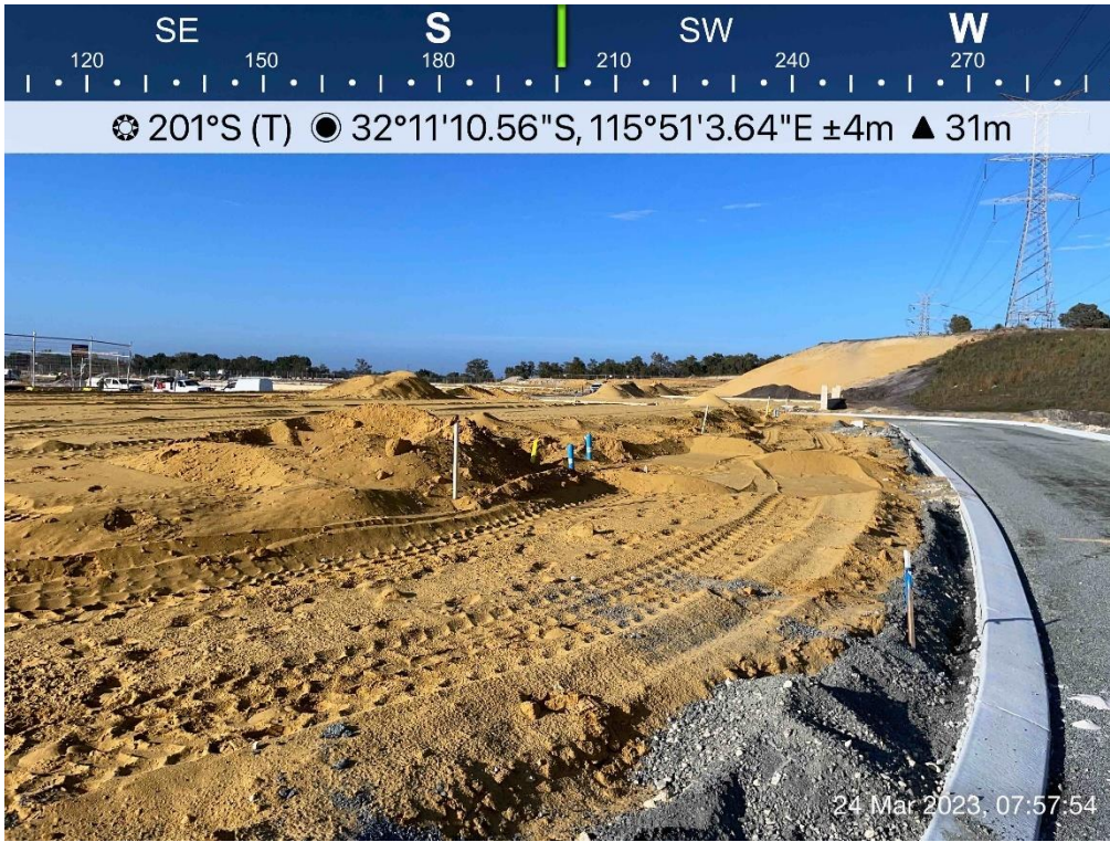
Plate 7: Installation of water reticulation within Stage 8
