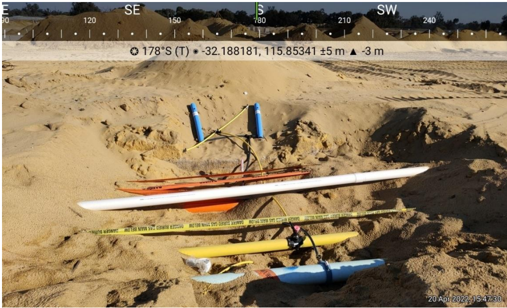
Plate 7: Installation of water reticulation within Stage 12.
