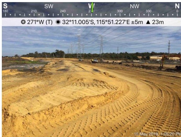
Plate 1: EAW under construction (east-west section)
